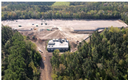
Groundworks nearing completion
