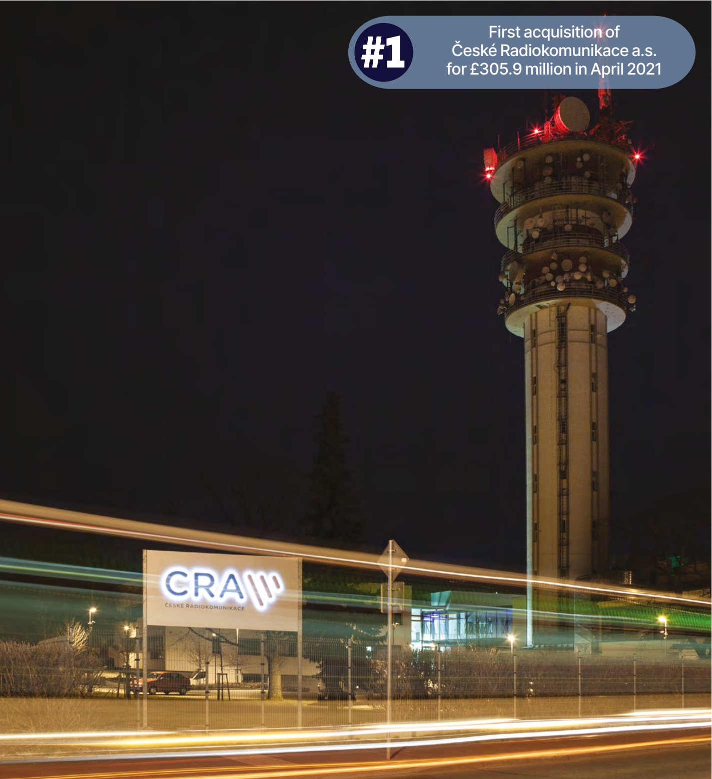
One of CRA's network of towers
