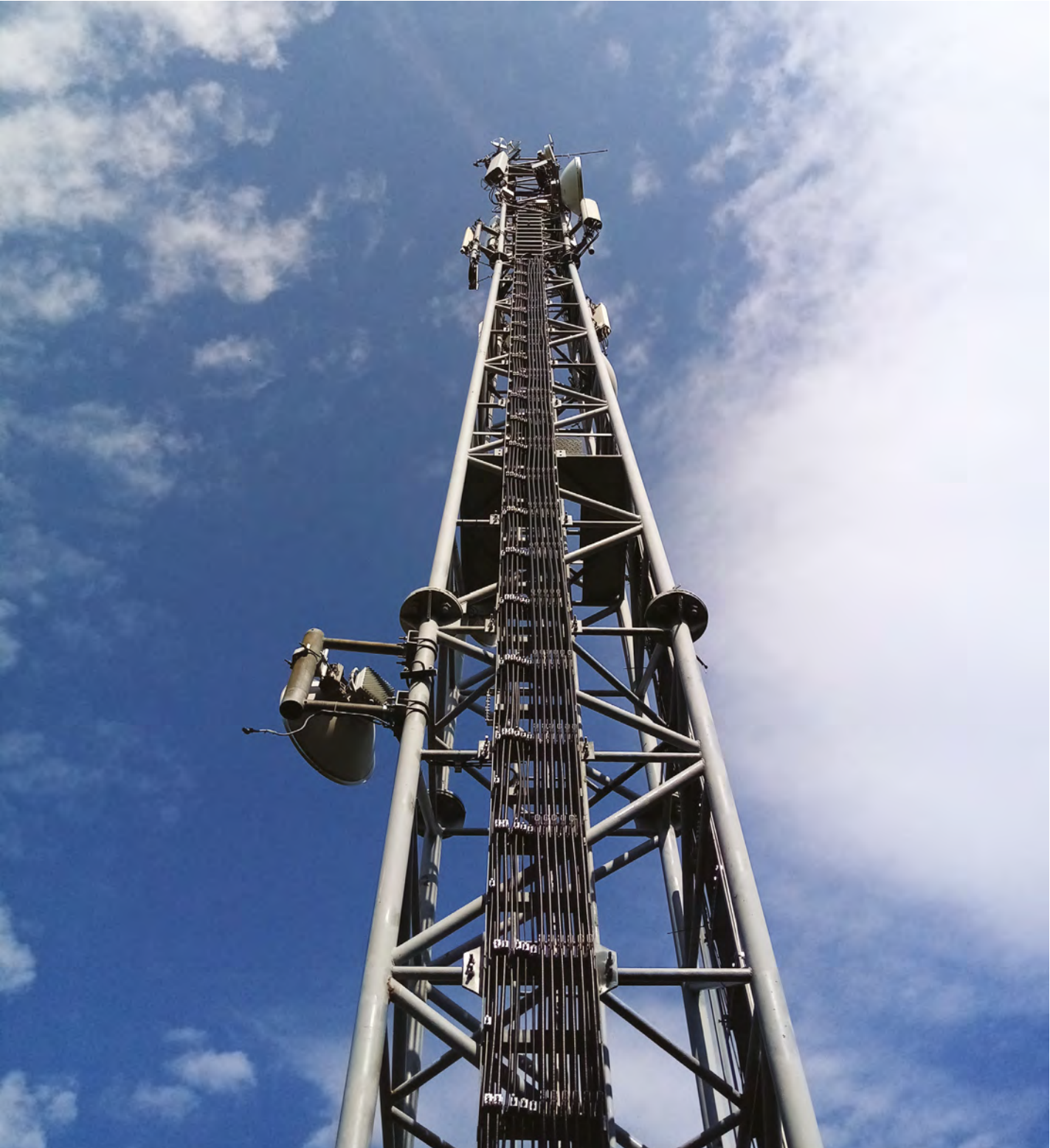
One of CRA's network of towers
